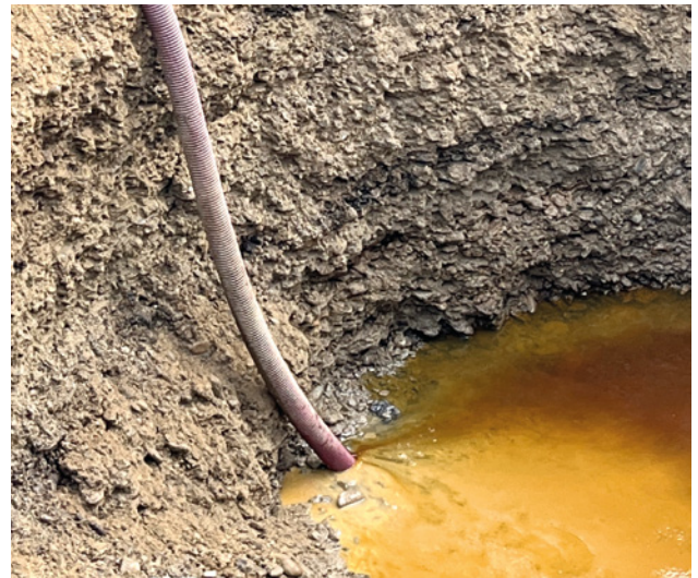
Pumping benzene from an excavation site
