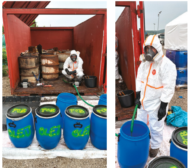
Repackaging and removal of waste from the site
