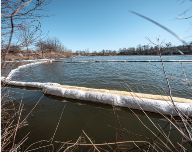
Prevention of benzene spreading on the water surface using sorption snakes
