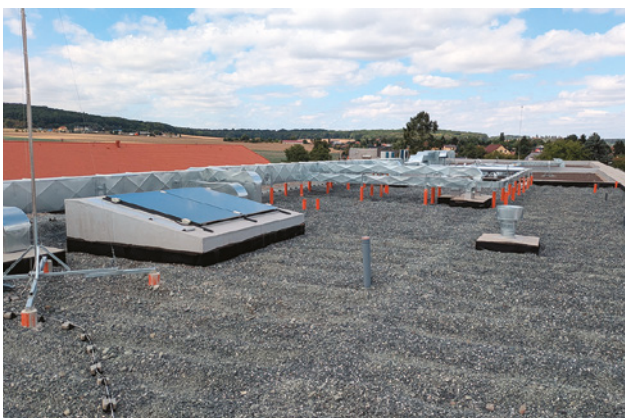
The rooftop constructed wetland before planting.
