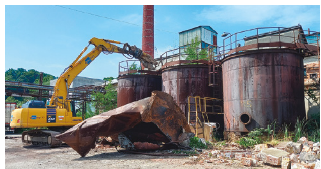
Demolition of tanks using hydraulic shears
