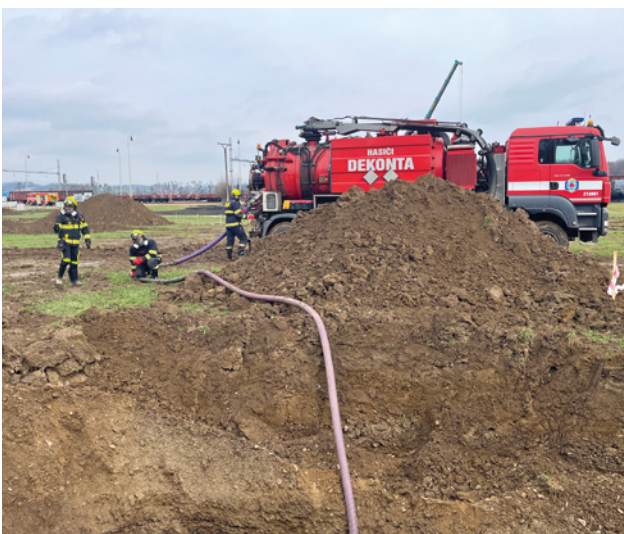
Benzene removal by a specialized team of firefighters Dekonta
